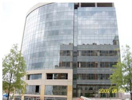
Figure 6: Curtain Wall System
