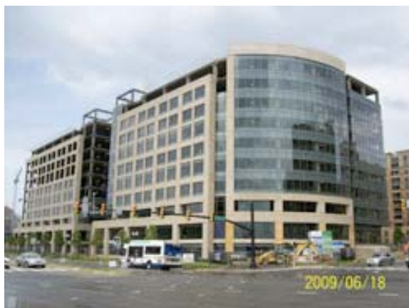
Figure 1: View from US Rte.1
